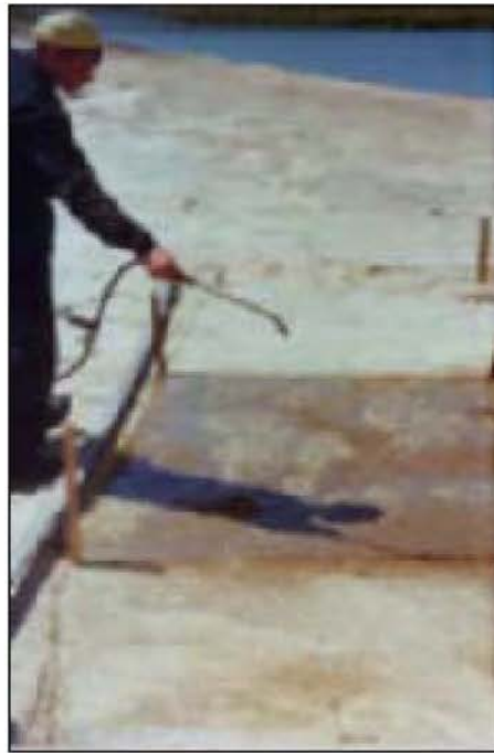
Fig. VII-54. The process of application of polymer coatings.
