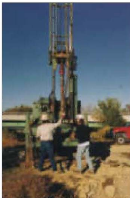
Fig. XIII-10. A drill rig is positioned prior to drilling a monitor well at a remediation site.
