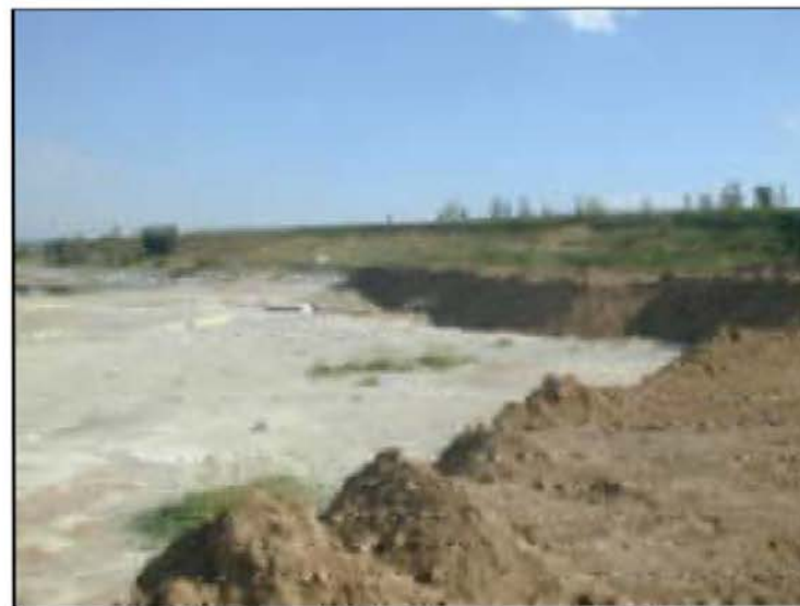
Fig. VII-53. Geotechnical failure and beach destruction after clay emplacement.
