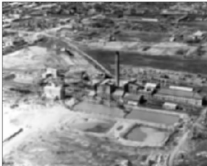
Fig. XIII-11. This mill, located near Grand Junction, Colorado, processed uranium ore from 1951 until 1970; three tailings ponds are visible in the foreground.
