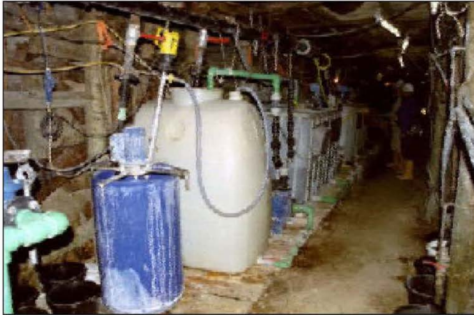
Fig. VI-49. View of the grout plant used for the preparation of the BaSO 4 forming solution.
