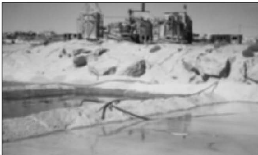
Fig. XIII-1. During the early years of processing uranium ore in the United States, liquid waste was piped to ponds where the liquid component evaporated, leaving fine sandlike tailings.
