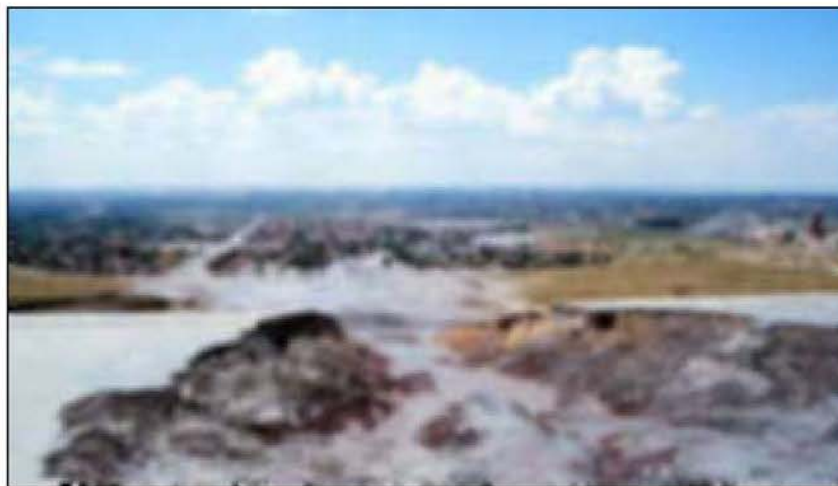
Fig.5. The Merriespruit (South Africa) tailings dam failure in 1994 [35].
